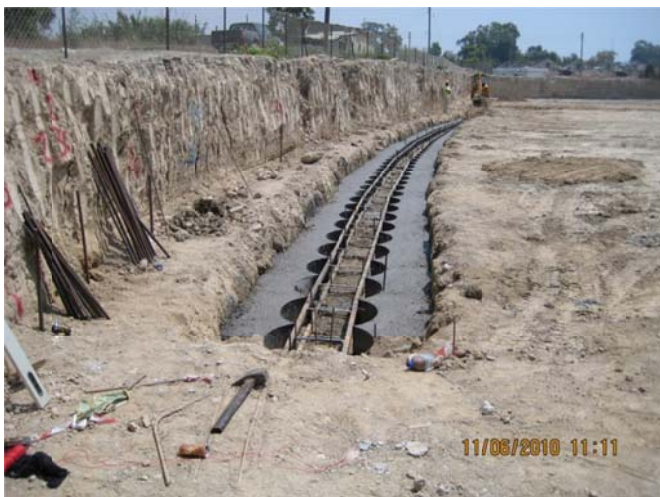
Figure 6 – Construction Stage 4 – Construction of secant pile wall
