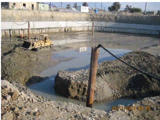
Figure 7 – Construction Stage 5 – Completion of excavation with dewatering
