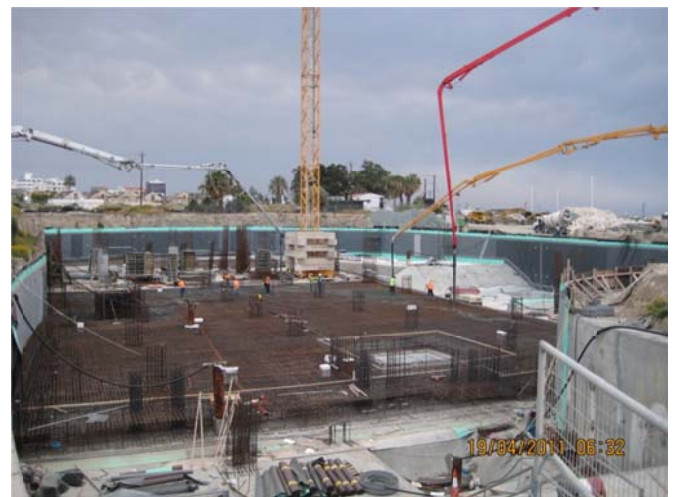
Figure 9 – Construction Stage 6 – Construction of raft foundation
